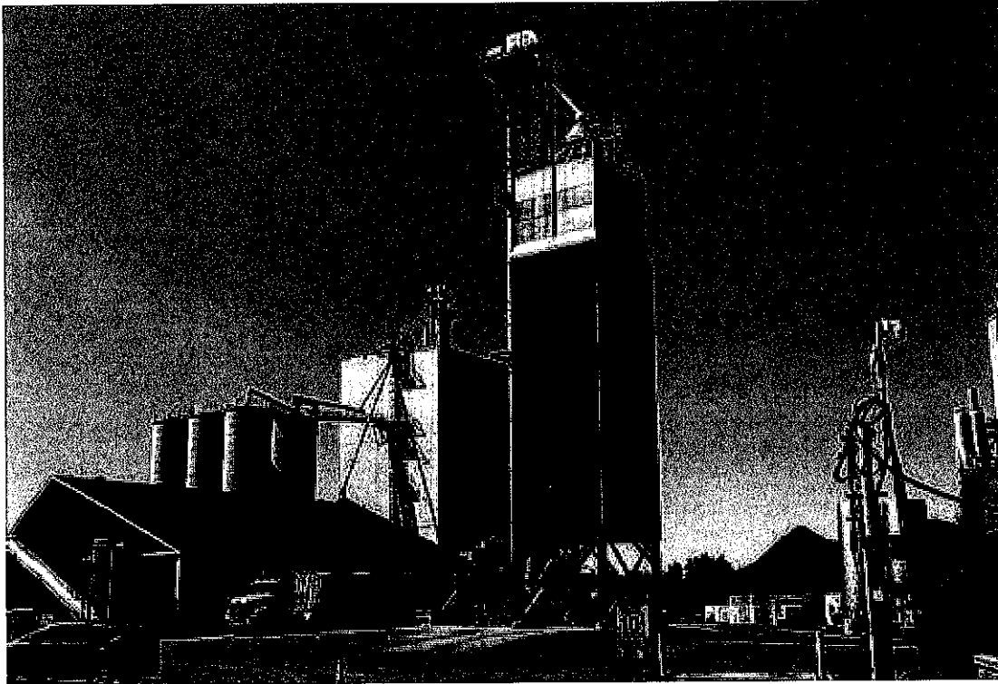
Figure 6. Existing fertilizer blending facility on site
